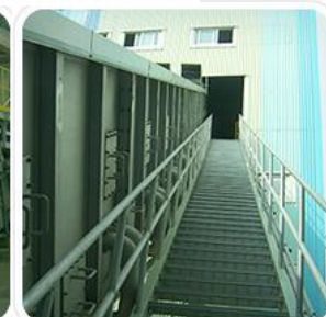
○ 보령화력 Dry-Type Bottom Ash System
