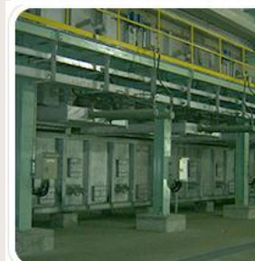
○ 보령화력 Dry-Type Bottom Ash System
