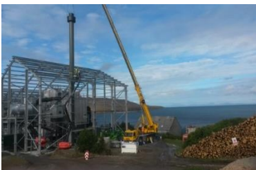
Erection of Stack on the Isle of Iskay
