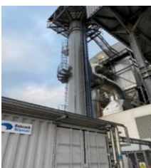
▷ Stack structural shell cleaned, superficial Corrosion removed and areas painted
