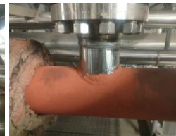
168mm Pressure nozzles changed out along with 25mm feedline
