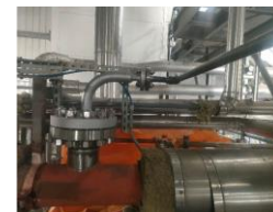
168mm Pressure nozzles changed out along with 25mm feedline
