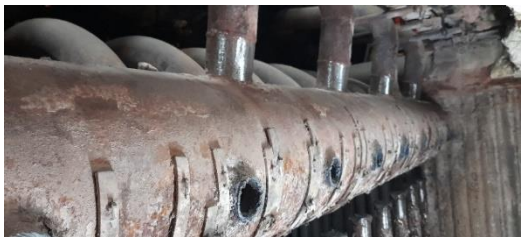
Header inside Boiler being Cut out
