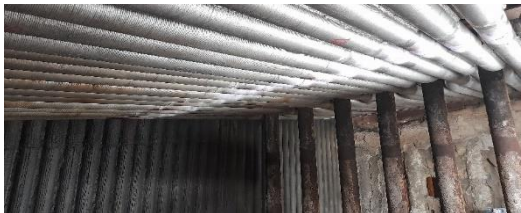
Header inside Boiler being Cut out
