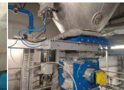
Slide Valve replaced
