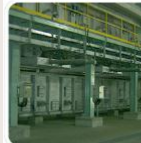
○ 보령화력 Dry-Type Bottom Ash System
