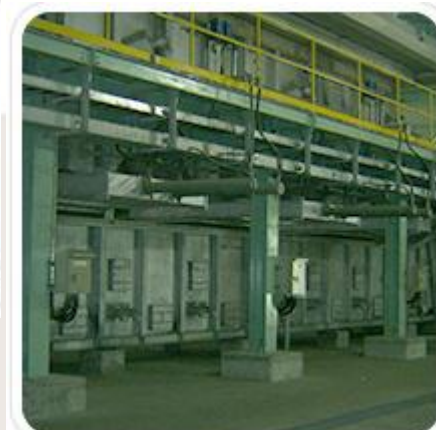
Dry-type Ash system at Boryeong Thermal Power Plant
