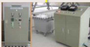
Control panel and high voltage panel
